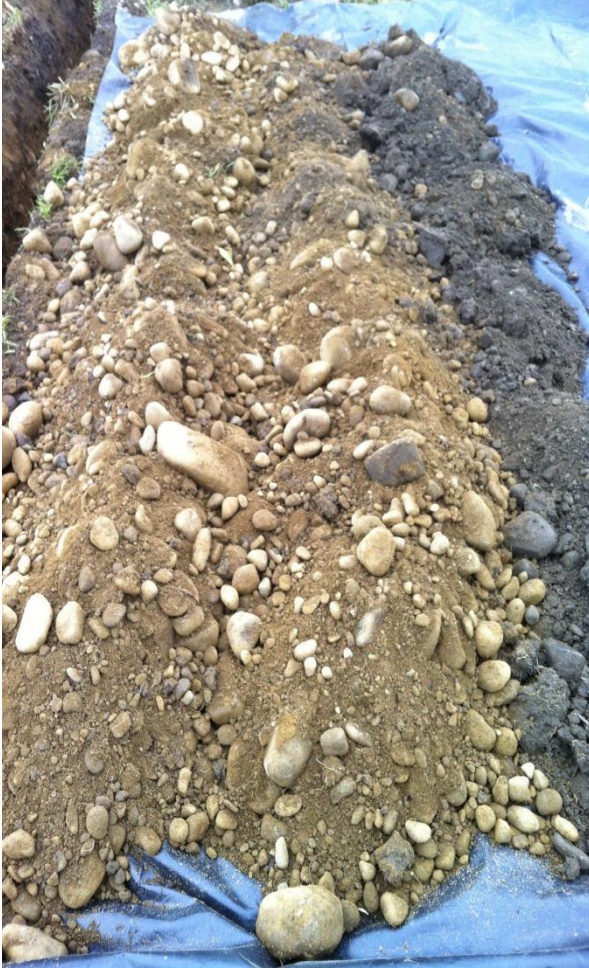
Soil removed and placed in three layers.
