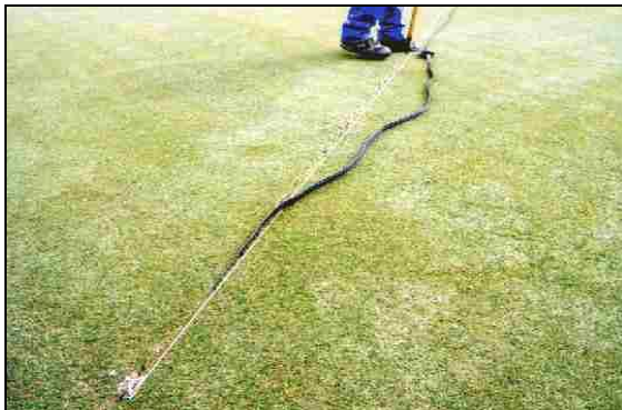
Run string line and cut a slit in turf
