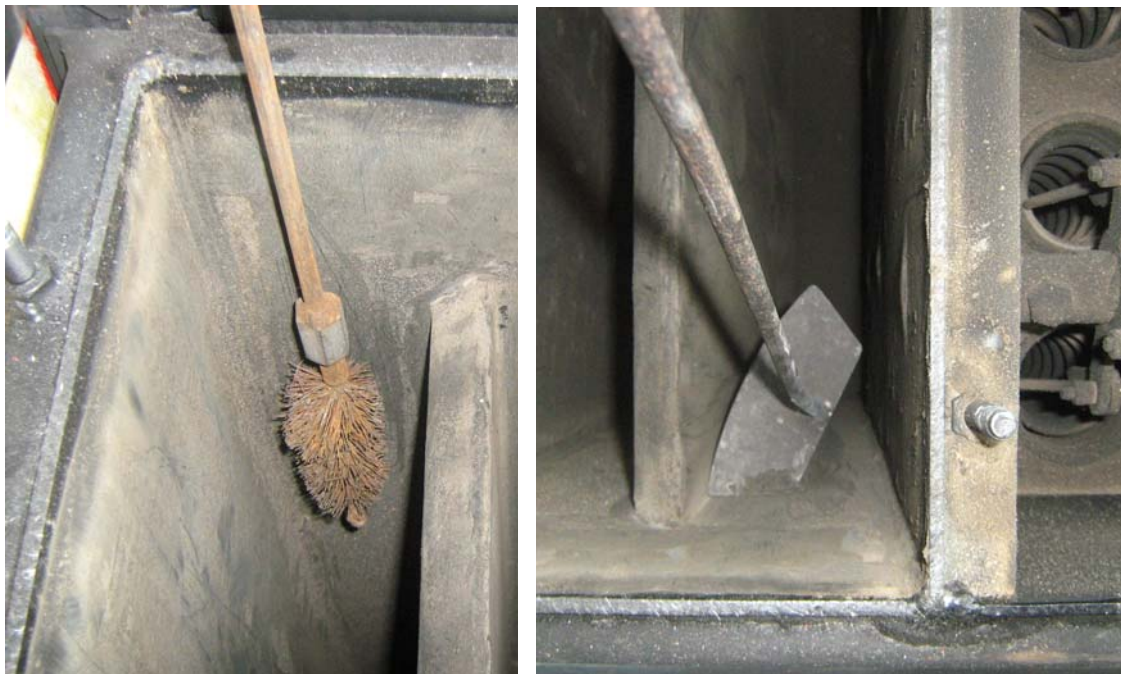
Figure 2.4. Brushing the ash layer of the heat exchanger surfaces;
