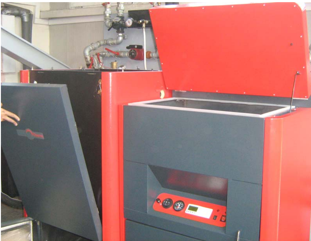
Figure 2.8. Detaching the front panel of the heat exchanger;
