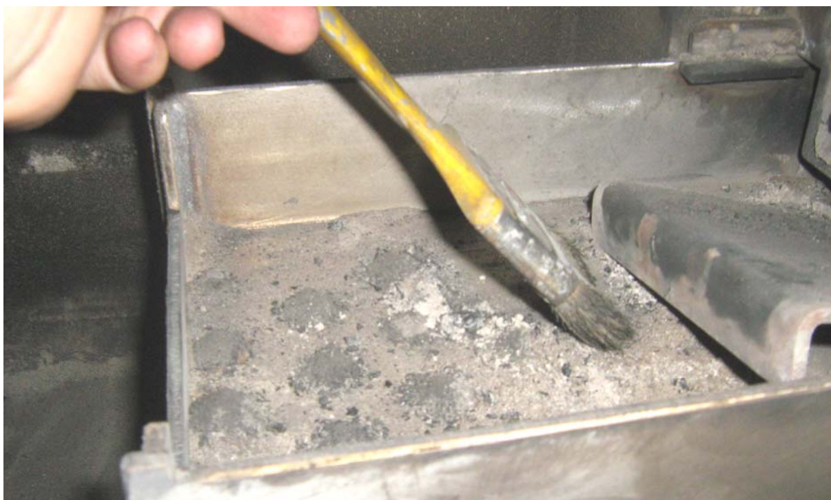
Figure 2.15. Cleaning the ash residue, fallen beneath the grate of the burner;
