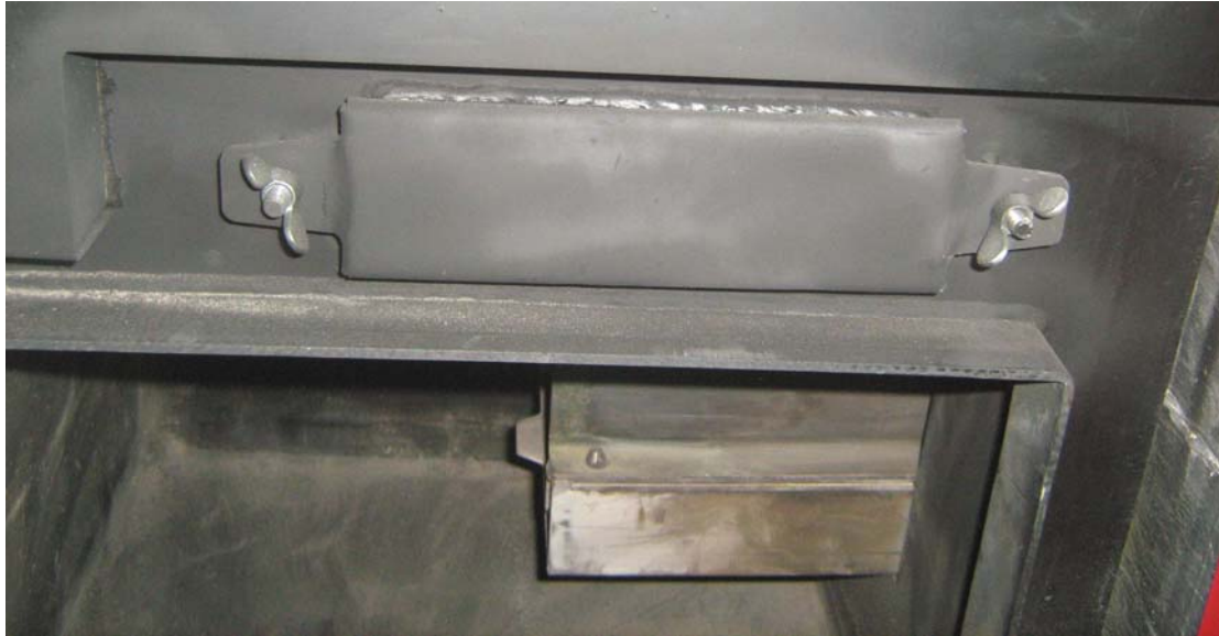
Figure 2.9. The lid of the secondary ash deposition zone is detached and the ash layer should be cleaned away;
