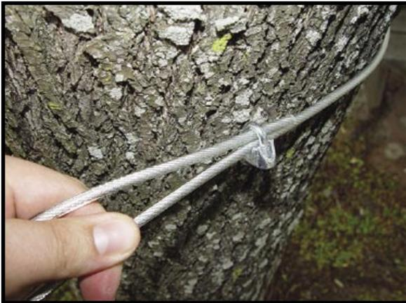
Pull the cable ends tight so that the Echo is tight against the tree or pole, then tighten the nuts on the cable clamp using the installation kit's nut driver, as shown in the figure below.
