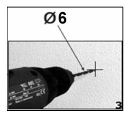
**3)** Using a drill bit with a 6 mm diameter, make holes in the wall on the positions that you have marked in step 2.
