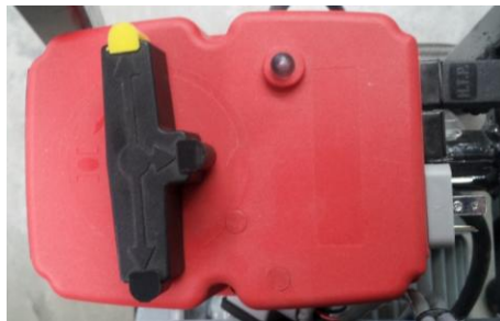
Figure 14 – Normally closed position
