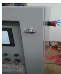
Figure 6b – Emergency stop button
