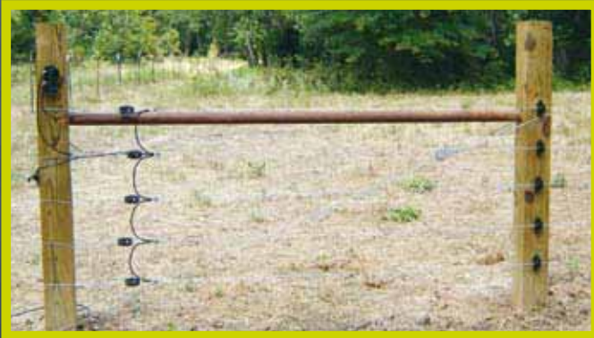
H brace for the start of a 5-wire fence
