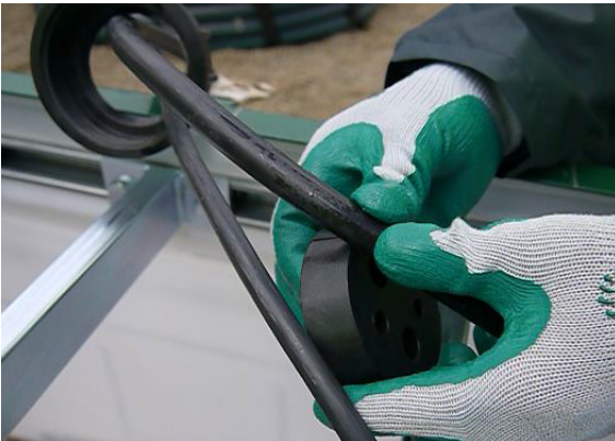
Figure 6: Tilt the Compression Disk to Insert Cables
