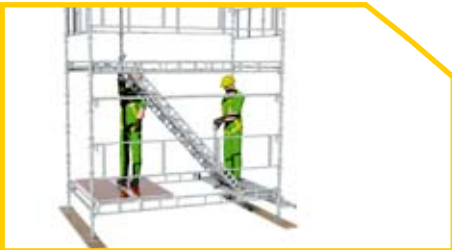
23 Install Guardrail posts in the upper and lower Landing Platforms.
