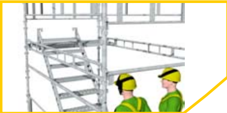
21 Stair flight is then lowered to meet the upper landing pushing it into position.
