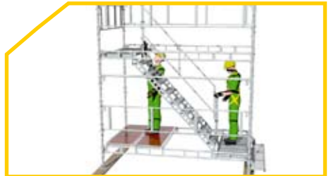
24 Install Stair handrail to Guardrail Posts ensuring that catches are fully secured.
