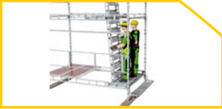
19 Stair flight is placed vertically into the pockets on the lower Landing Platform. Stair should be fitted in a clockwise ascent.
