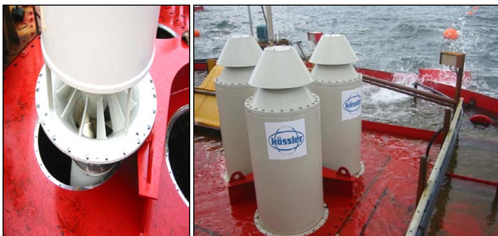
Fig. 4.13 Installation of draft tube and installed turbines.
