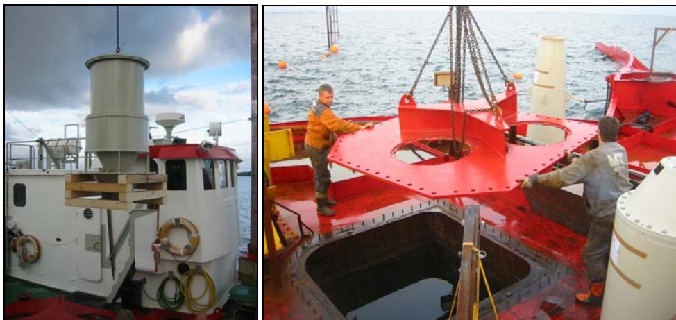
Fig. 4.11 Unloading of turbine centre and installation of floor plates section (runner & guide vanes)
