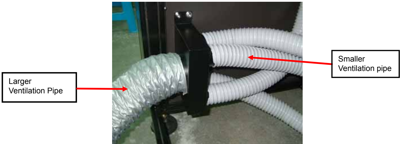
(Figure 5- 14 Connecting the Exhaust System))
