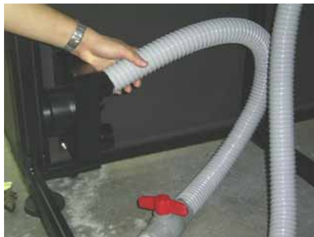
(Figure 5- 11 Connecting the Exhaust System)
