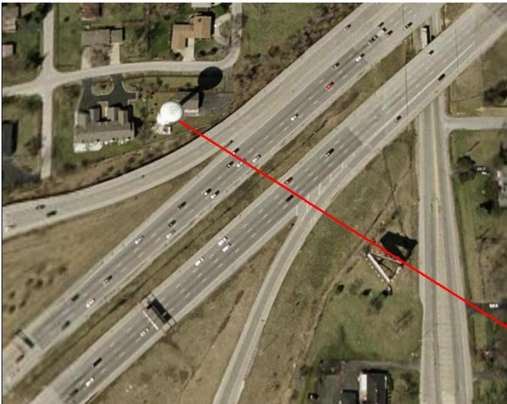
Figure 4 – Microwave link, aerial view
