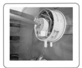
5. Turning the knob in the centre of the pressure sensor, turn to the Camfil recommended final pressure drop. For sensor location, see also the "Schematic diagram of the junction box" (above).
