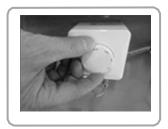
To switch the fan off, turn the potentiometer anticlockwise until a click is heard.
