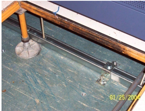
Fig. 2.2.1 Subfloor bracing
