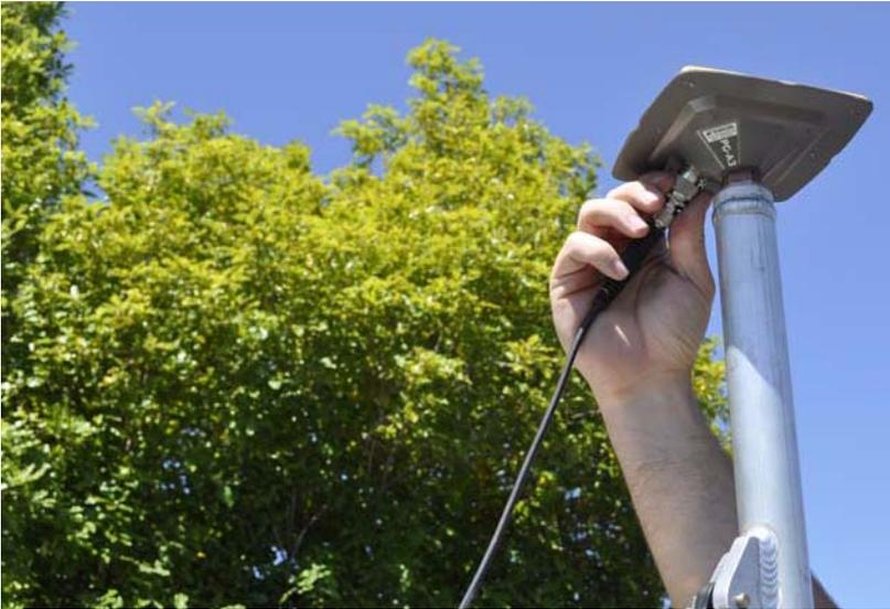
Figure 2-25. GPS Antenna Cable to GPS Antenna
