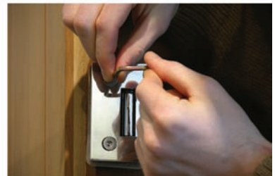
Hex tool tightens hinge
