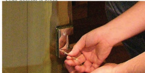
Tighten hinge with hex tool
