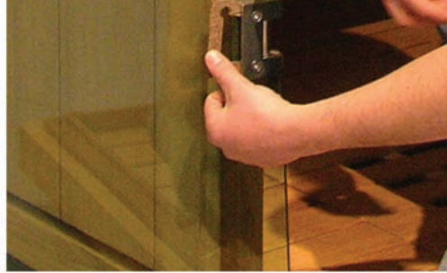
Slide gaskets in place
