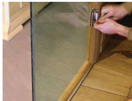
Tighten hinges while door rests on spacer
