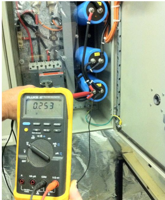
Figure 14 - Voltage measurement of a capacitor
