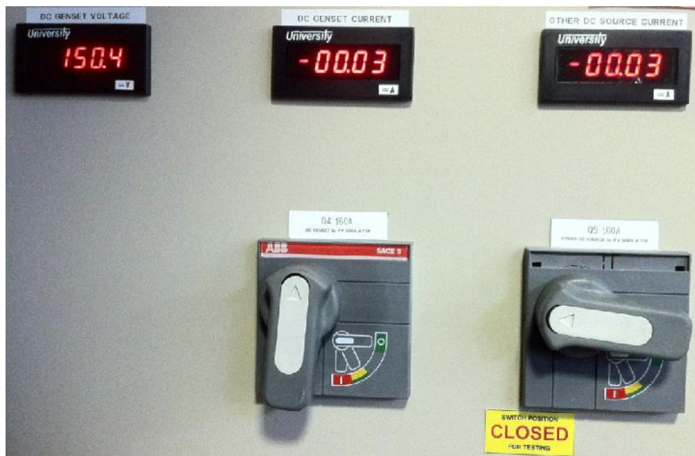
Figure 10 - PV Simulator Input/DC Genset Output Panel
