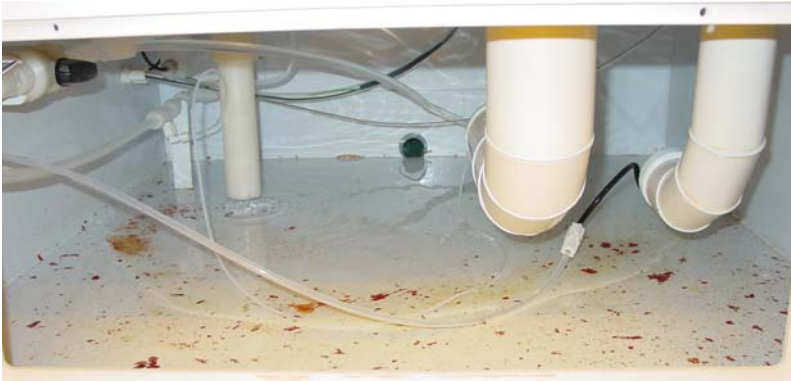
Figure B6. This is the sump where the water drains from the sink. Do not throw resist in this sink! Resist dissolved in developer is ok. NO SOLVENTS!!! (Solvents will dissolve the hood).
