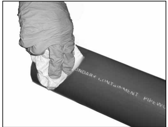
Clean Secondary with Acetone
