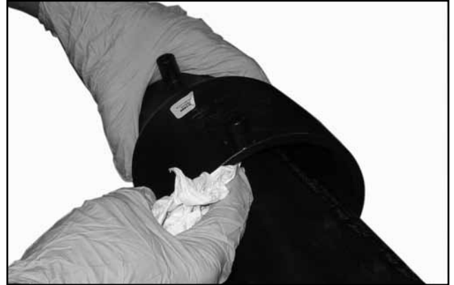
Clean Inside of Secondary
