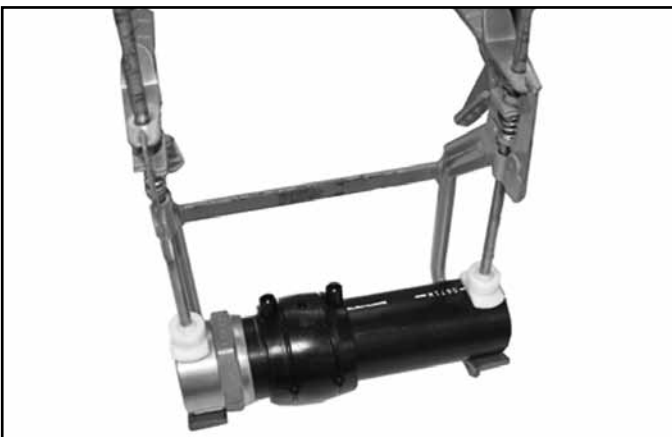
Straight Clamp Installed
