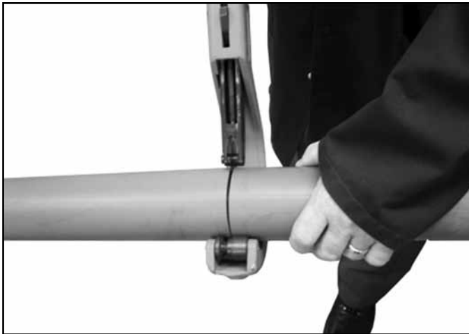
Cut Secondary Pipe
