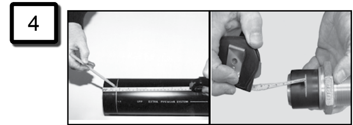
4 Measure and mark pipe to indicate correct insertion depth into fusion fitting.
