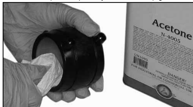
Clean Weld Coupler with Acetone
