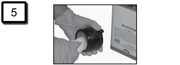
5 Clean bore of the welding coupler with Acetone.
