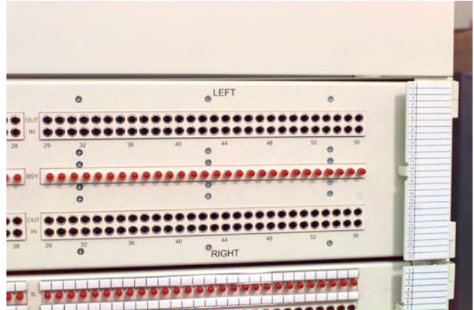
Figure 8 - Patch Panels
