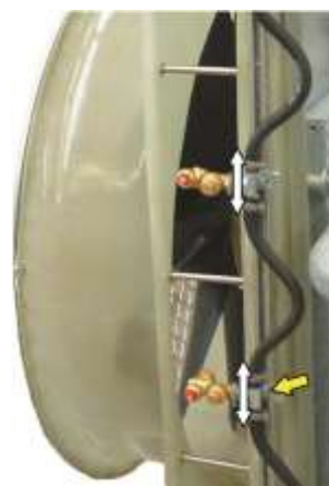
Rectifier with adjustable nozzles
