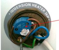
Press the silver immersion button on the Samsung remote controller; this will force the immersion heater on. Check immersion heater works properly, Measure the current drawn by the heater; it should be 12-13 Amps.
