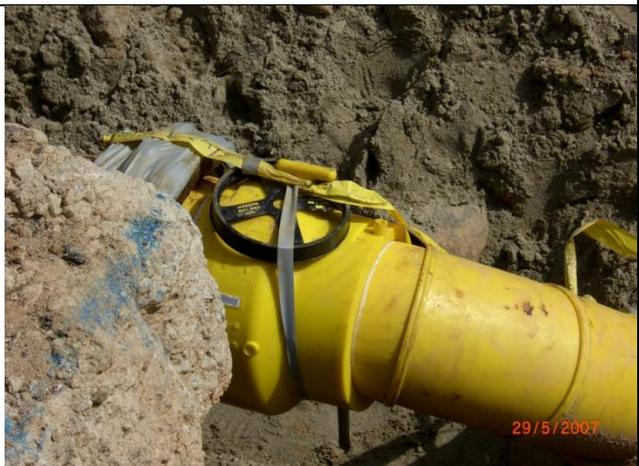
F: A Mini-Marker installed on a gas pipe
