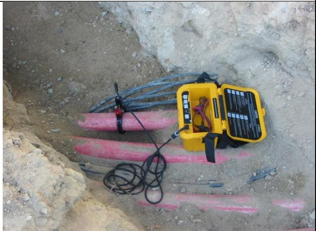
D: A signal clamp is used on an exposed cable duct
