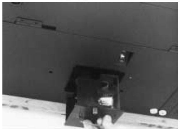
Removing the lamp; lamp door was removed.
