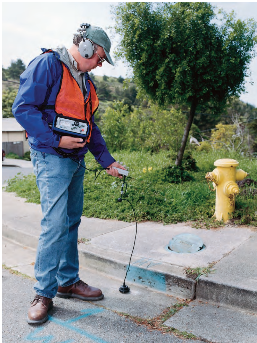
Figure 4-9 Leak Pinpointing Over a Hydrant Line
