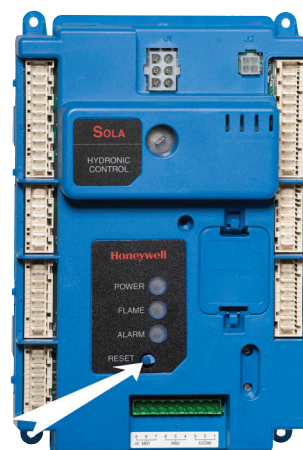
Figure 34. Reset Button on Controller
