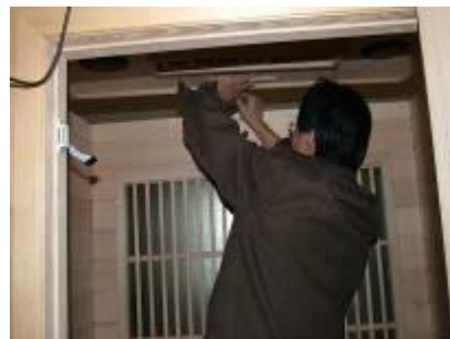
FIG-13 Lead the heater wires through the holes in the roof
