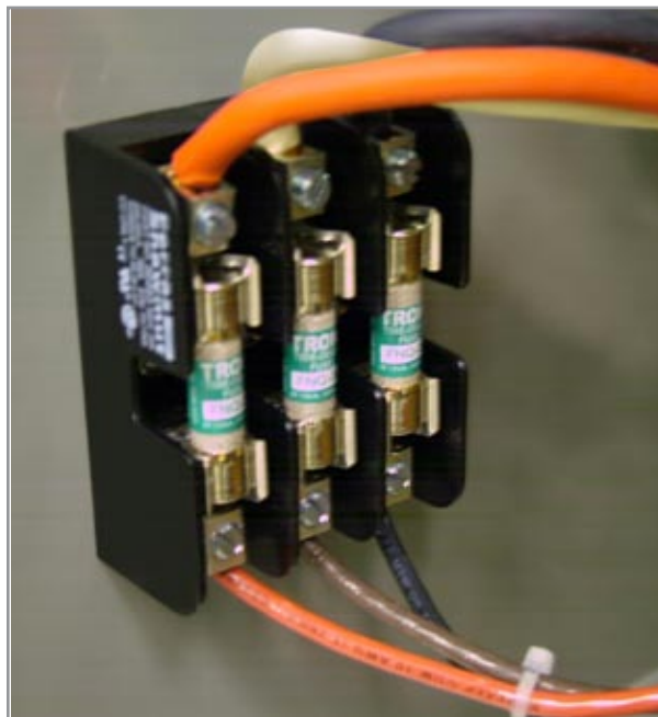
Figure 2.10.1 Replaceable Fuses
