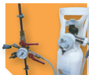
Supplying the network with backup cylinder
