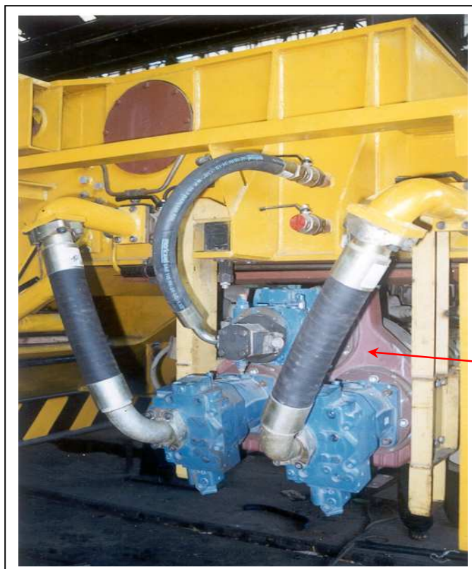
Pump distributor gearbox
