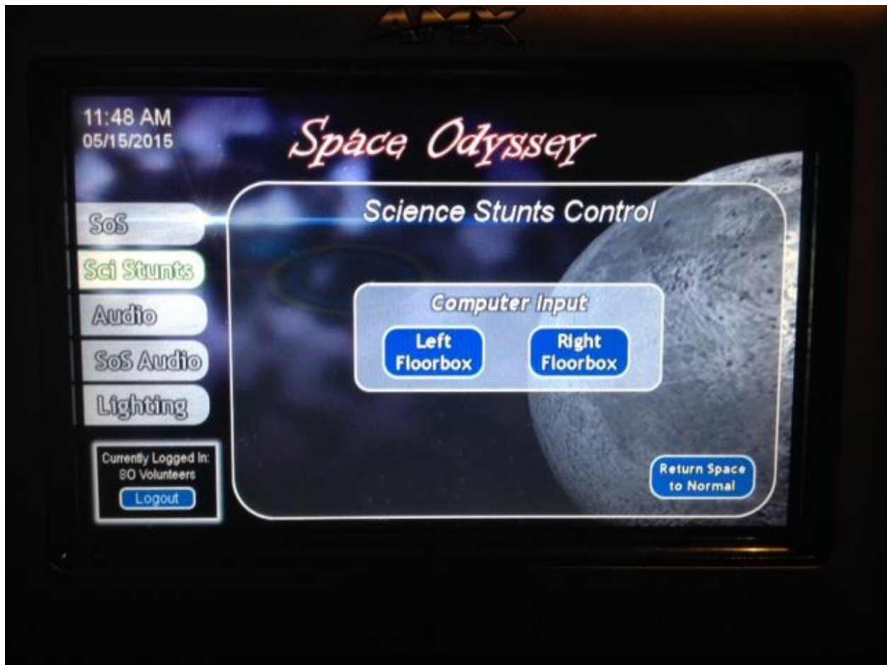
Figure 9 showing the “Sci Stunts” screen on the AMX panel which allows you to send the laptop/iPad image to the drop-down screen adjacent to the SOS. Note the “Return Space to Normal” button at the bottom right which, when tapped, will let you reset the space once you’re done using it.
