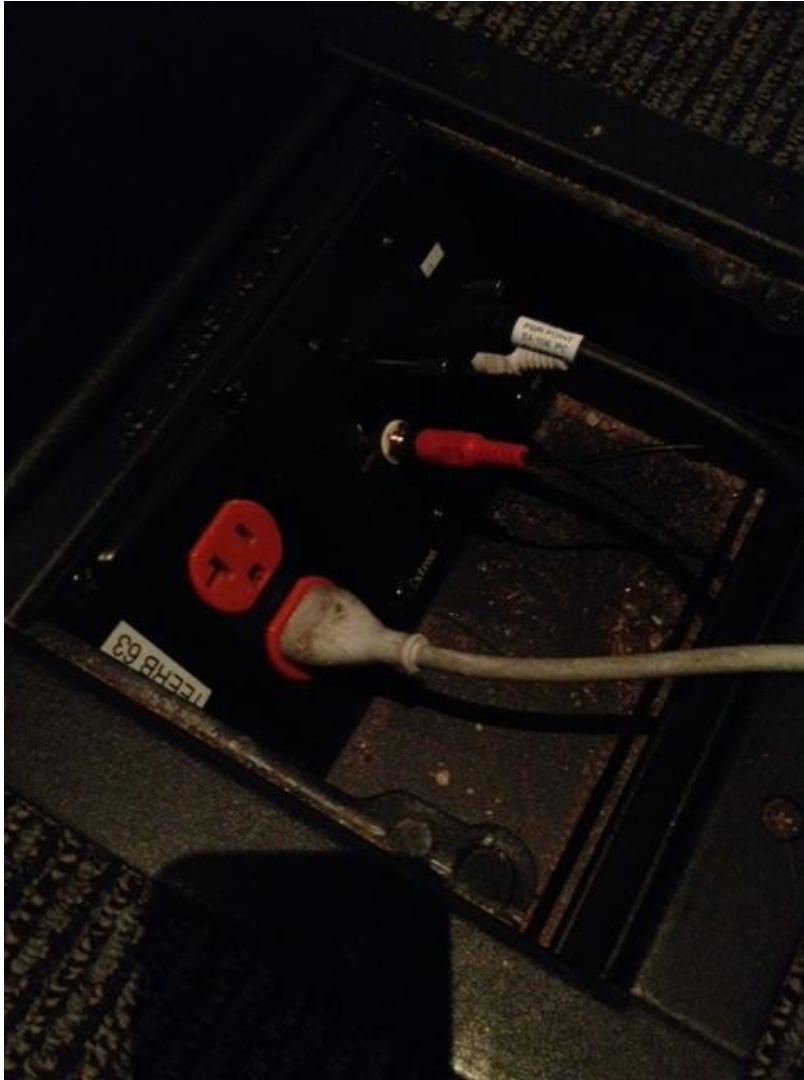
Figure 3 : Shows the power plug and audio plugs inserted into the outlets in the floor box.
