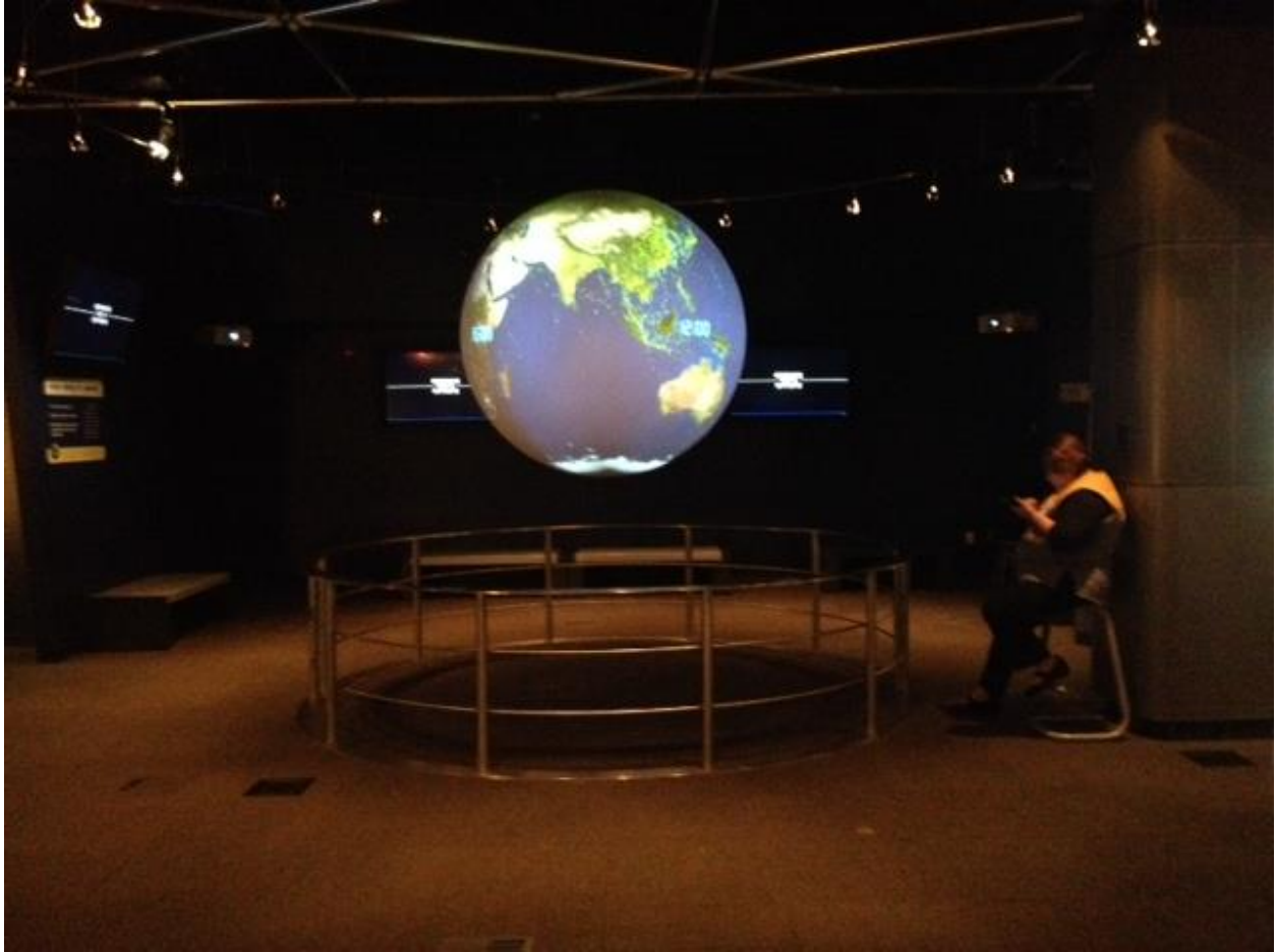
Figure 1 shows SOS with back screens plus left floor box near the lower left section of the guardrail and right floor box at the base of the column. The AMX panel is on the column on the right and is mounted on the side facing the SOS.
