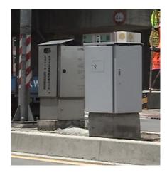
**Traffic Signal Controller UPS (T.S.C.UPS)** is consists of two major parts, which including UPS system and Battery system.
