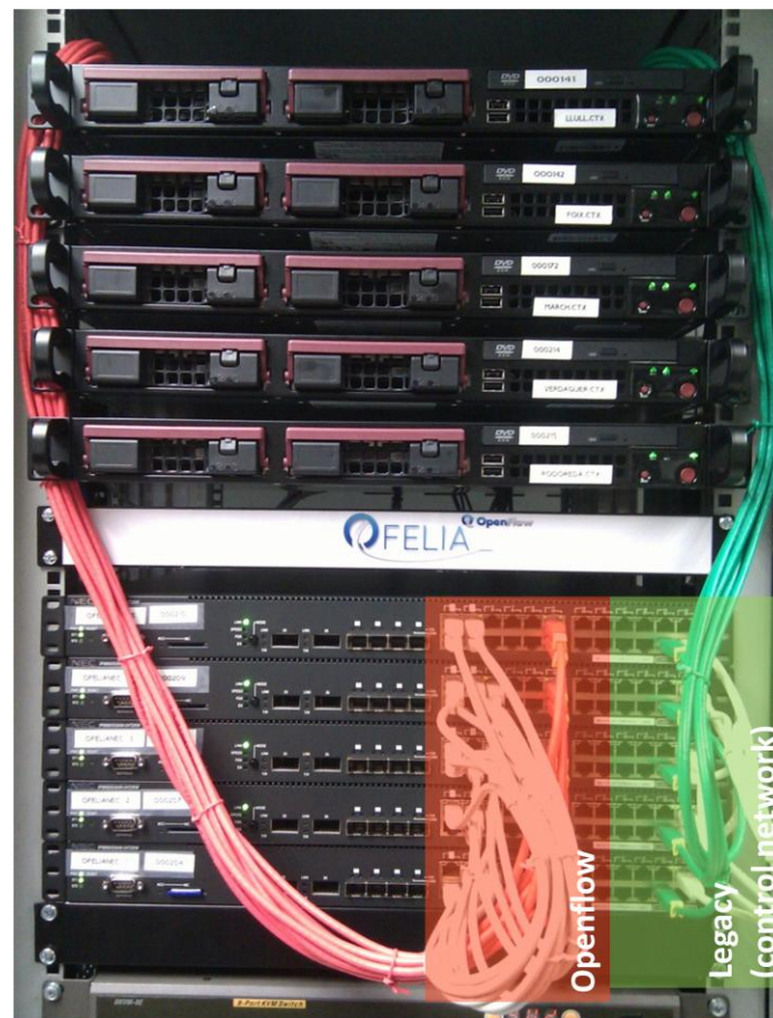
Figure 18: Equipment in place (NEC switches only)
