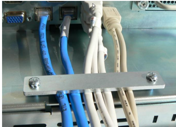
Cable Securing Bar Installed
