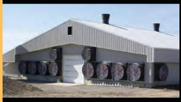
In a tunnel ventilation building, use the Supra to control tunnel fans and curtains, pit fans, wall fans, ceiling inlets, and heaters. The Supra can close ceiling inlets or switch off wall fans when changing to tunnel mode.
