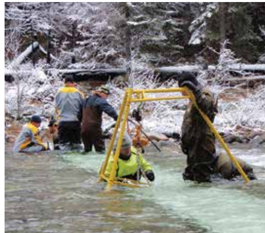
Biomark Stout™ antenna installation. East Fork of the South Fork of the Salmon River, Idaho.
