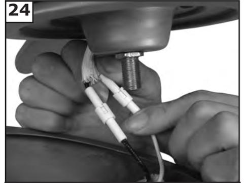
**24** Connect white wire from fan to white wire from light fixture. Then plug black wire from fan to black wire from light fixture.
