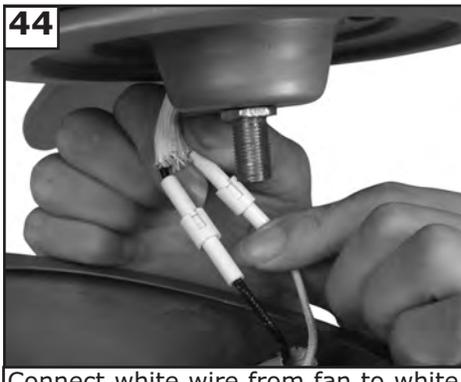
44 Connect white wire from fan to white wire from light fixture. Then plug black wire from fan to black wire from light fixture.
