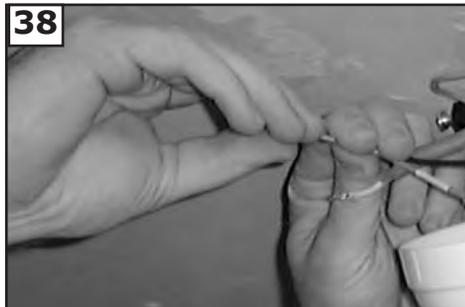
**38** Make wire connections to power source using wire nuts provided. Make sure that no filaments are outside of the wirenut. After making the wire connections, the wires should be spread apart with the grounded conductor and the equipment-grounding conductor on one side of the outlet box and ungrounded conductor on the other side of the outlet box.
