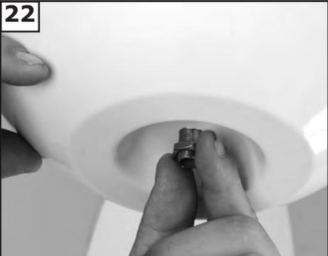
**22** Install light plate over all thread and use nut provided to secure in place.
