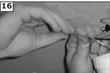
**16** Make wire connections to power source using wire nuts provided. Make sure that no filaments are outside of the wirenut. After making the wire connections, the wires should be spread apart with the grounded conductor and the equipment-grounding conductor on one side of the outlet box and ungrounded conductor on the other side of the outlet box.
