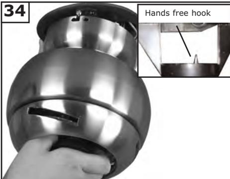
**34** Hang fan from mounting bracket by the hands free hook into a closed hole on the edge of the Canopy. Note: For Canadian mounting refer to Step #10.
