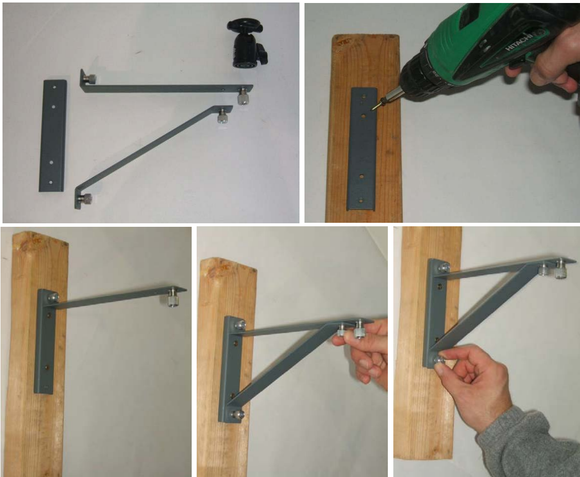
Figure 12 Thermal Camera Bracket Assembly Procedure
