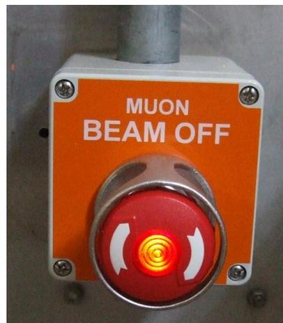
Figure 3: A muon beam off button
