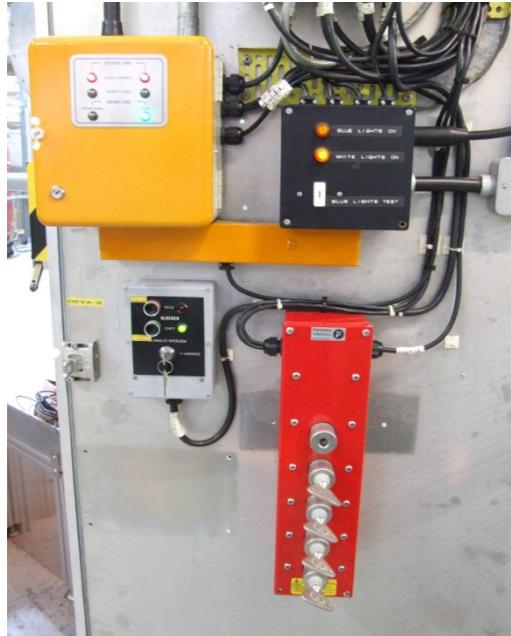
**Figure 2: Interlock key box, master switch, and main door lock.**
