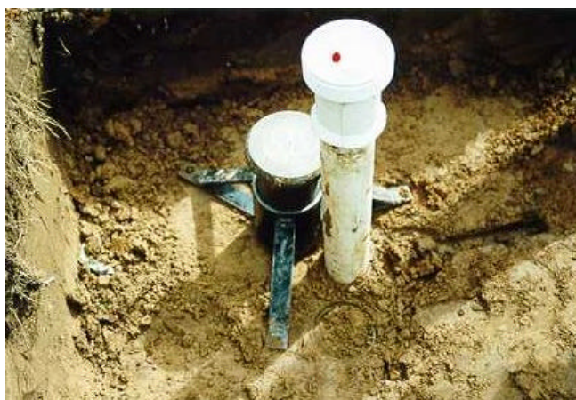
Photo 6. Placing top on ring extension ready to hit with mallet
