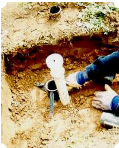
Photo 5. Placing ring extension on top of ring
