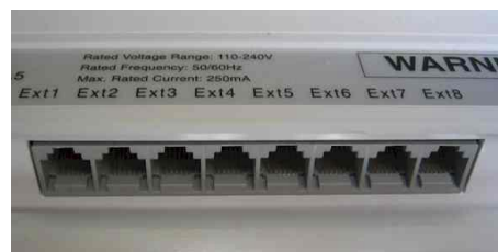
The 8 RJ12 extension ports of the Premier PABX
