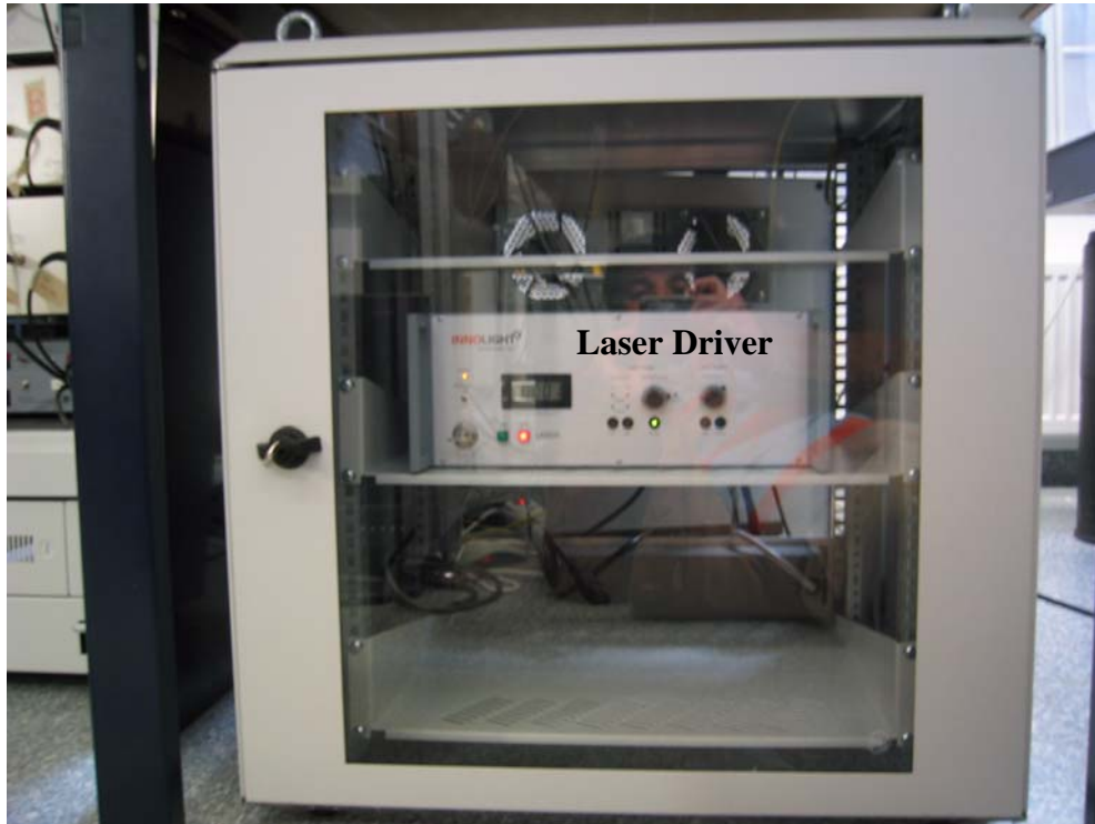
Figure 34 Metrology Cabinet 3, hosting the laser driver
