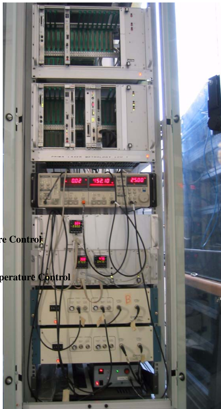
Figure 32 Metrology Cabinet 1 during testing in Garching
