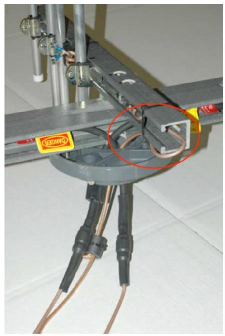
There is a cable access hole in the lower end of the mast. Guide the antenna cables into the top of the hollow mast. Thread the cables through the lower cable access.
