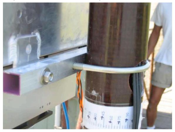
Mount the antenna to the top of the mast.
