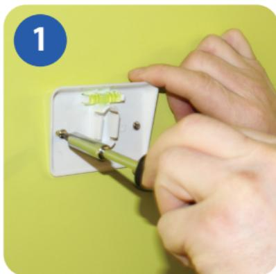
1 Attach the wall mounting bracket to a suitable wall using the fittings supplied and the built in level.
