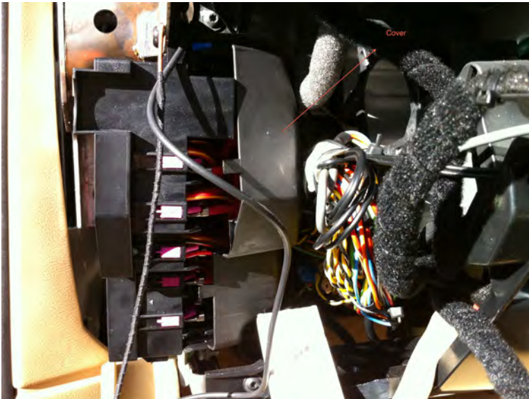
Picture 24 – red arrow shows the fusebox back cover
