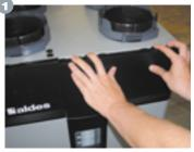
Press the two buttons on the top of the unit and remove the panel on the top right.
