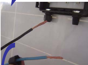
Insert the cable to the junction box, pay attention of the positive and negative
