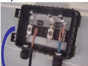
Fixed the cables ◦
