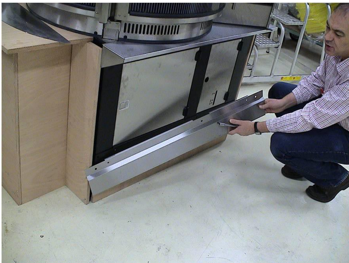
Connect the plinth for the under frame.
