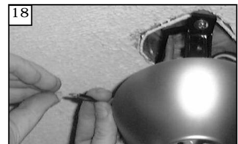
18 Make wire connections to power source using wire nuts provided. Make sure that no filaments are outside of the wirenut. After making the wire connections, the wires should be spread apart with the grounded conductor and the equipment-grounding conductor on one side of the outlet box and ungrounded conductor on the other side of the outlet box.
