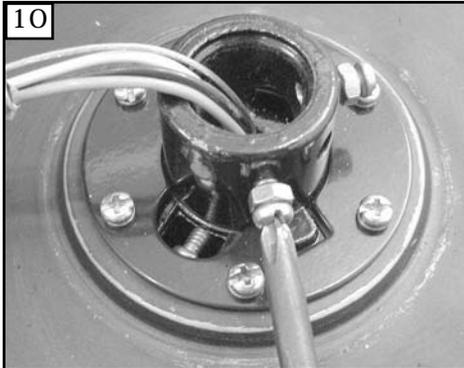
10 Loosen 2 screws and remove pin with keeper for downrod, yoke cover, and canopy to fit in yoke of fan.
