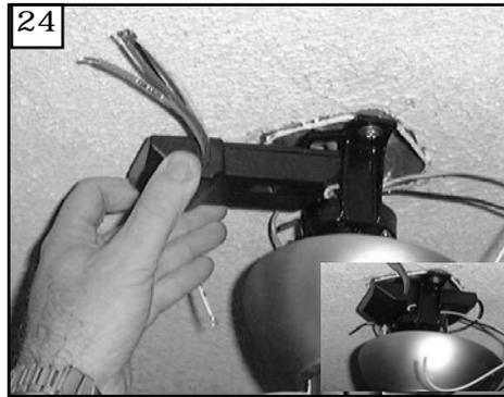
24 Install remote receiver by sliding into opening in the Mounting bracket. Make sure that the dip switches on the Transmitter and the Receiver are set to the same position. See Fig 42 for remote operation
