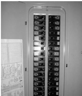
Before you begin installing the fan, Switch power off at Service panel and lock service disconnecting means to prevent power from being switched on accidentally. When the service disconnecting means cannot be locked, securely fasten a prominent warning device, such as a tag, to the service panel.
