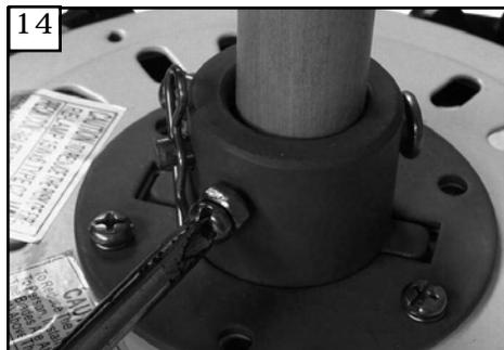
Tighten 2 downrod set screws and lock nuts.
