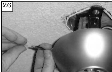
26 Make wire connections to power source using wire nuts provided. Make sure that no filaments are outside of the wirenut. After making the wire connections, the wires should be spread apart with the grounded conductor and the equipment-grounding conductor on one side of the outlet box and ungrounded conductor on the other side of the outlet box.
