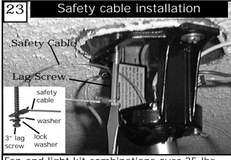
23 Fan and light kit combinations over 35 lbs, in both flush and downrod mode the safety cable must be installed into the house structure beams using the 3" lag screws, washers, and lock washers, provided. Make sure that when the safety cable is fully extended the lead wires are longer than the cable and no stress is placed on the lead wires.
