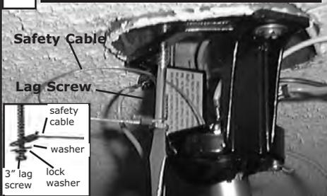
Fan and light kit combinations over 70 lbs, in both flush and downrod mode the safety cable must be installed into the house structure beams using the 3" lag screws, washers, and lock washers, provided. Make sure that when the safety cable is fully extended the lead wires are longer than the cable and no stress is placed on the lead wires.
