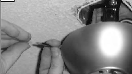
Make wire connections to power source using wire nuts provided. Make sure that no filaments are outside of the wire nut. After making the wire connections, the wires should be spread apart with the grounded conductor and the equipment-grounding conductor on one side of the outlet box and ungrounded conductor on the other side of the outlet box.
