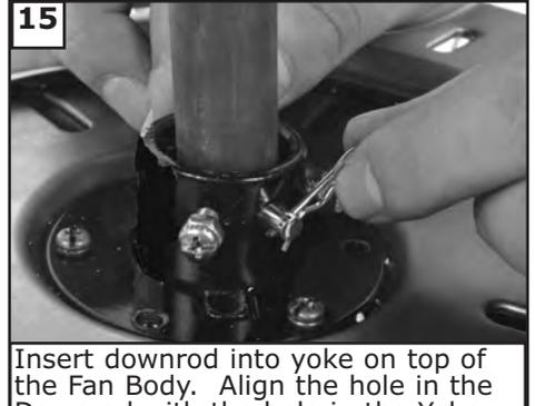
15 Insert downrod into yoke on top of the Fan Body. Align the hole in the Downrod with the hole in the Yoke. Insert the Pin through the Yoke and Downrod until the point appears on the other side. Install the Keeper Pin
