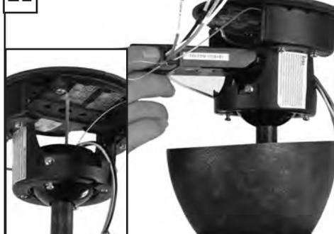
Install remote receiver by sliding into opening in the Mounting bracket. Make sure that the dip switches on the Transmitter and the Receiver are set to the same position.
